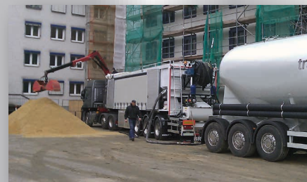
Because of the horizontal production system, the installation can be reloaded during the production process
