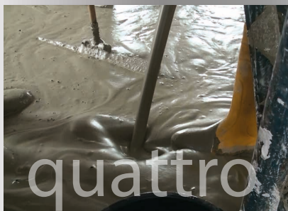
The Quattro version of the S3.17T XL has a foam-generator that can produce foam and inject it into the liquid mortar for producing foam mortar.
